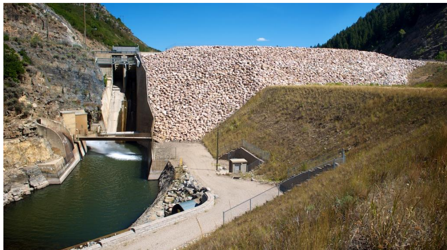
Figure 3. Outlet works of Pineview Reservoir
