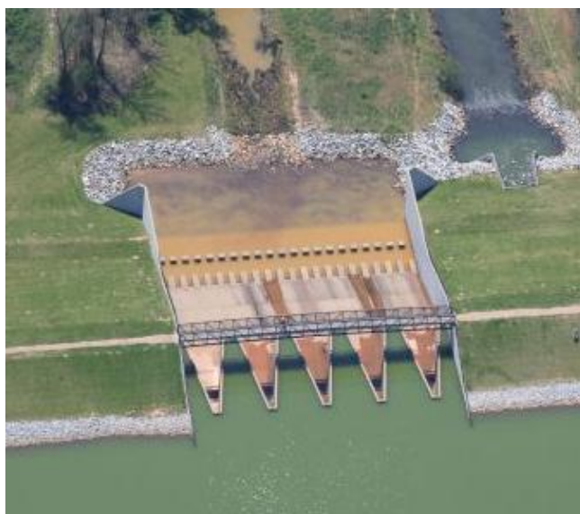
Figure 1 - Example of a Labyrinth Weir
