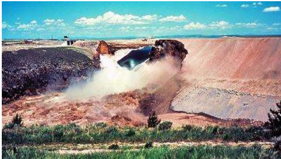
Figure 1. The Teton dam during the failure.
