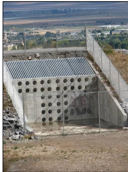
Figure 8. The outlet structure for the Logan Dry Canyon detention basin. Not visible is the single outlet culvert. (Photo Courtesy of David Rosenberg)
