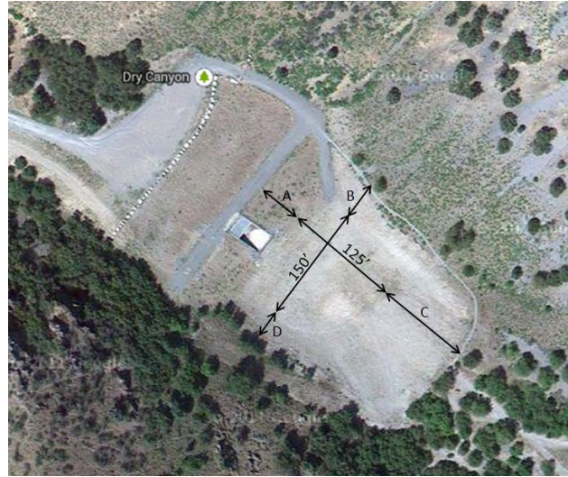
Figure 7. An aerial view of the existing detention basin at the mouth of Dry Canyon. The bottom of the basin (125'x150') is level ground. The sides A, B, C, and D are sloped 1:2, 1:2, 1:5, and 1:1, respectively. All dimensions given are approximate.
