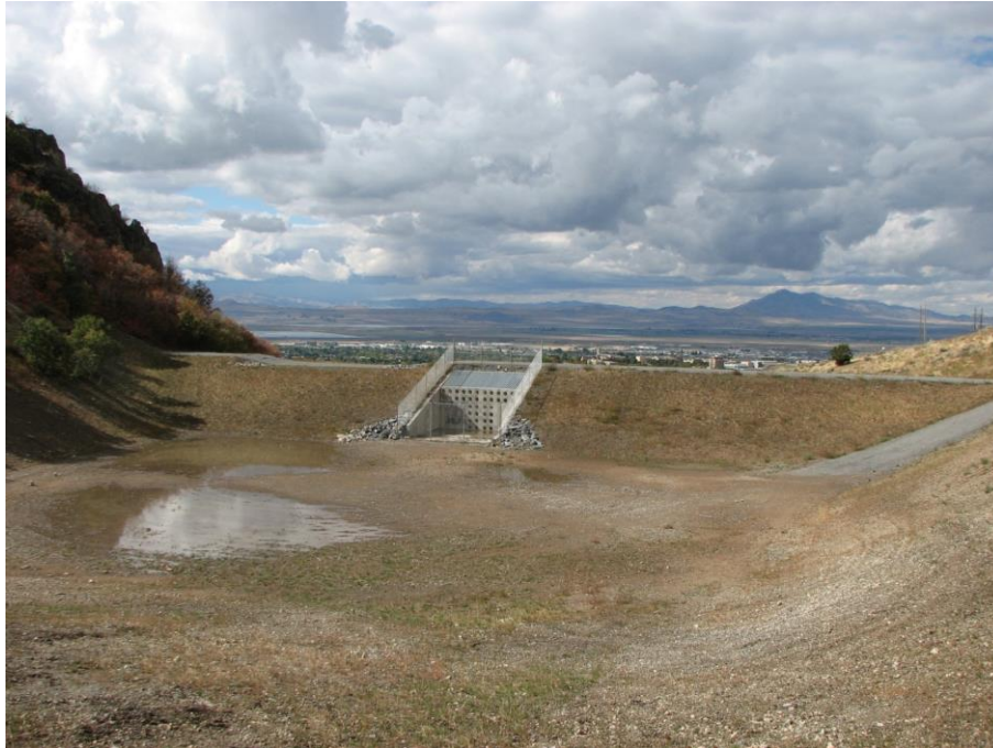
Figure 2. Logan Dry Canyon Detention Basin (Photo Courtesy of David Rosenberg)
